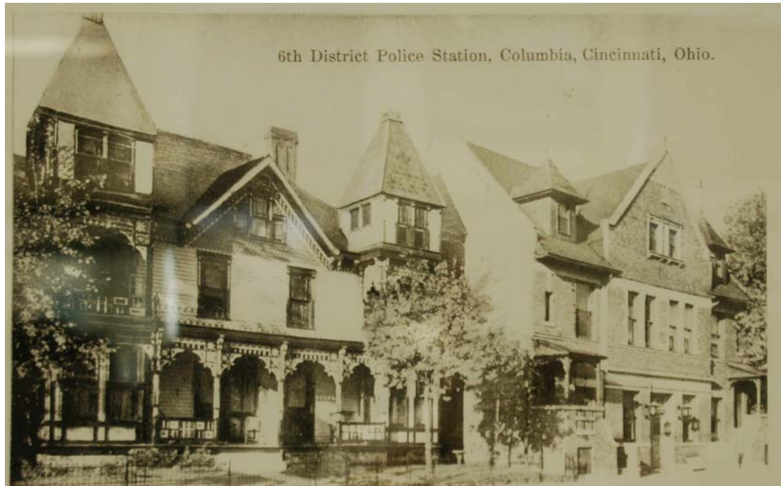
DISTRICT 6, 3855 EASTERN AVENUE, USED UNTIL THE 1950'S WHEN A NEW STATION WAS BUILT AT 3295 ERIE AVENUE
