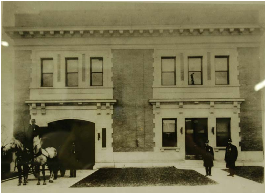
DISTRICT 3, WARSAW AVENUE, ORIGINALLY BUILT AS DISTRICT 9, IT WAS RENAMED DISTRICT 3 IN 1927, REMAINS IN USE 2006.
